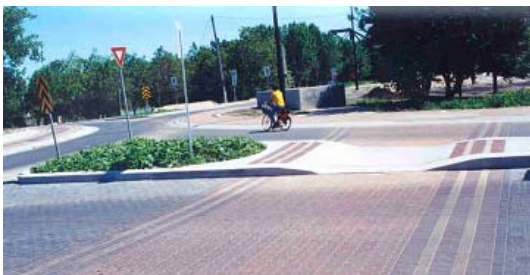
Texture and colour differences on a walkway enhances wayfinding for pedestrians.
