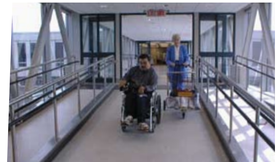
Weather protected walkways provide an accessible transition from outdoors to businesses and services .
